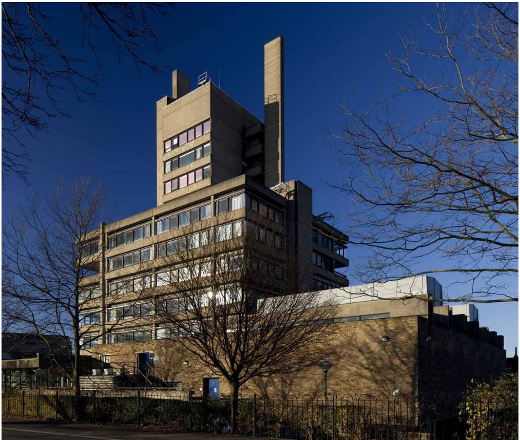
Figure 5. Charles Wilson Building, University of Leicester, Denys Lasdun & Partners, built 1964–7. This was the first to be built of Lasdun's sequence of university buildings largely constructed and clad in specially designed concrete components cast off-site, and tied into an in-situ concrete core. (Photograph by Barnabas Calder.)
