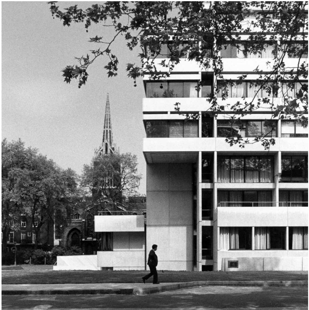
Figure 7. The School of Oriental and African Studies (SOAS), library extension, Denys Lasdun & Partners. Part of the University of London redevelopment on site from 1969. Comparison with UEA and the Charles Wilson building shows the variations in corner details, depth of window positions and proportions. After the Charles Wilson building the others make a clearer expression of the slab-like perimeter columns which free the floor-plate to be partitioned non-structurally. (Lasdun Archive/RIBA Library Photographs Collection.)
