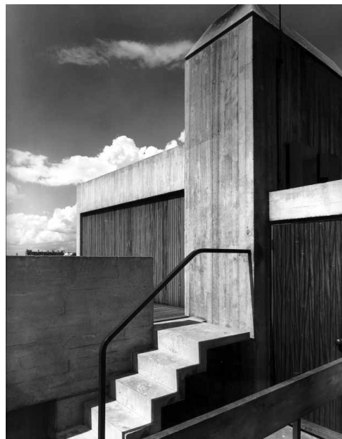
Figure 11. Flats at 26, St James's Place, London, Drake & Lasdun of Fry, Drew, Drake & Lasdun, completed by Denys Lasdun & Partners, 1958–61. Above the granite, brick and bronze of the luxury flats below, the penthouse roof-garden of the client allowed the tougher Corbusian vocabulary of exposed concrete to emerge. (Lasdun Archive/RIBA Library Photographs Collection.)
