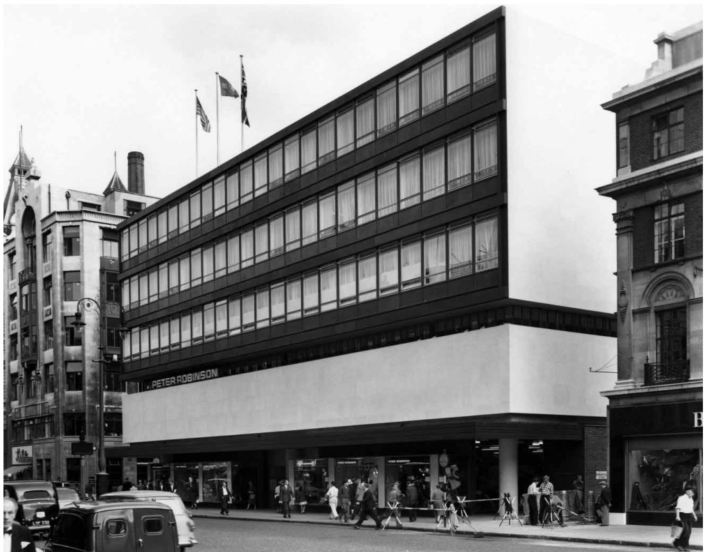
Figure 13. Peter Robinson department store, The Strand, London, 1957–9 (demolished), Drake & Lasdun of Fry, Drew, Drake & Lasdun. The upper façade is clad in a specially made pressed-bronze system, unlike Lasdun's later dark-brown buildings, which exploited the increasing availability of bronze-anodised aluminium. (Henk Snoek/RIBA Library Photographs Collection.)
