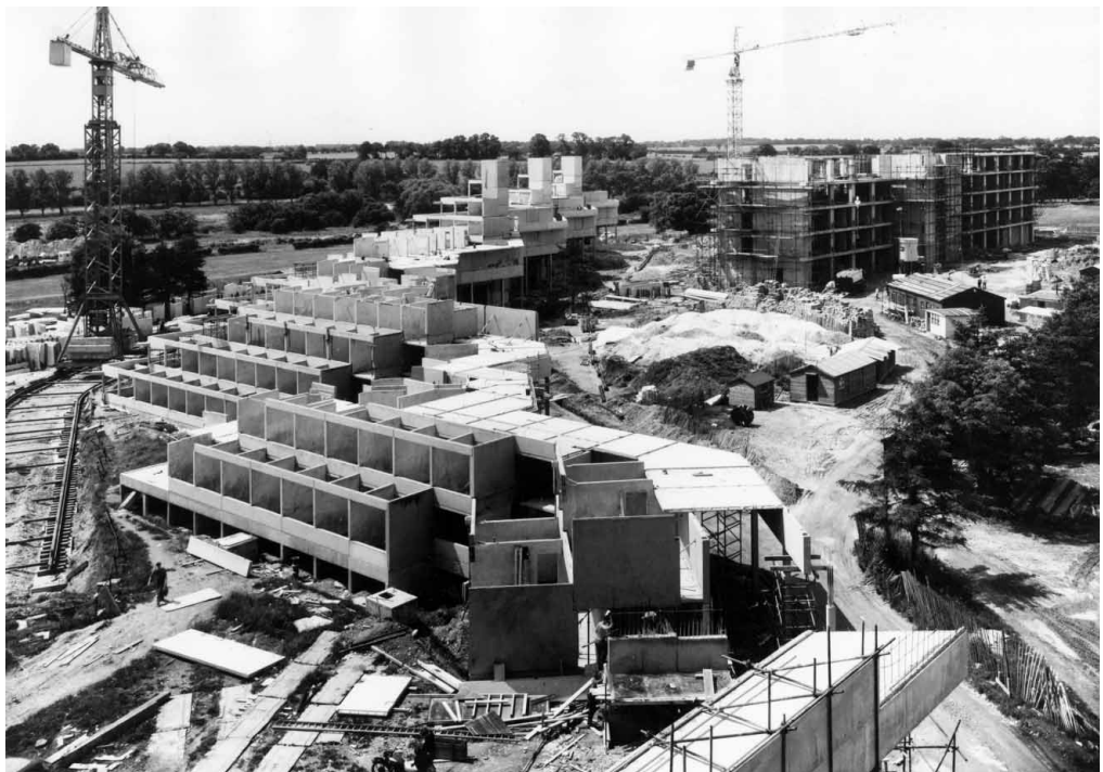
Figure 1. University of East Anglia (UEA), Denys Lasdun & Partners, built 1965–70. Construction photograph showing the student residences being assembled by a crane on tracks, carrying pre-cast components from the casting yard at the centre of the site. On the right the Teaching Wall is being constructed from a pre-cast system tied into in-situ cores. (Lasdun Archive/RIBA Library Photographs Collection.)
