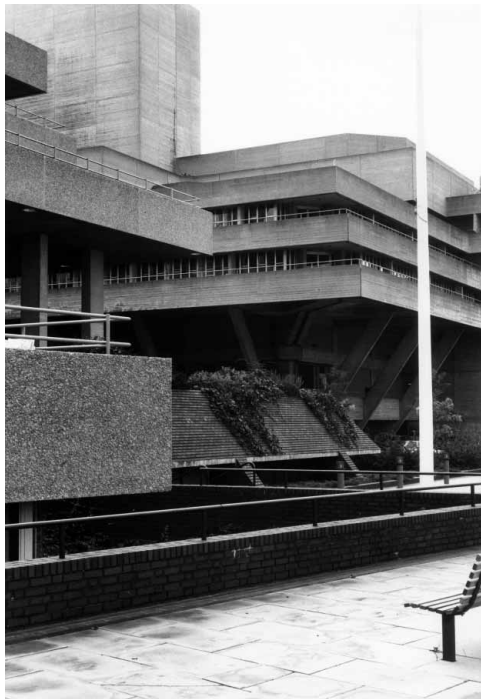
Figure 21. IBM Central London Marketing Centre (left), Denys Lasdun, Redhouse & Softley, 1983. Although in its use of terraced decks, blue engineering bricks and concrete, and in its careful massing, Lasdun's IBM was designed as the ideal neighbour for his masterpiece, the National Theatre, its concrete is not in fact the same. The use of pre-cast panels with exposed aggregate demonstrates his move away from exposed in situ in the later 1970s and 1980s. (Lasdun Archive/RIBA Library Photographs Collection.)
