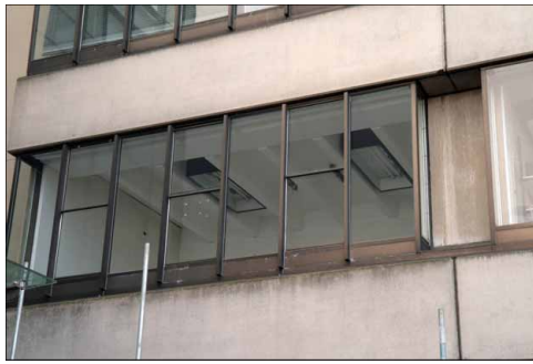
Figure 9. A detail of the Teaching Wall at the University of East Anglia (UEA), c. 2008, showing the good condition of the off-site pre-fabricated concrete, well-detailed and well-made to resist weathering. (Photograph by Barnabas Calder.)
