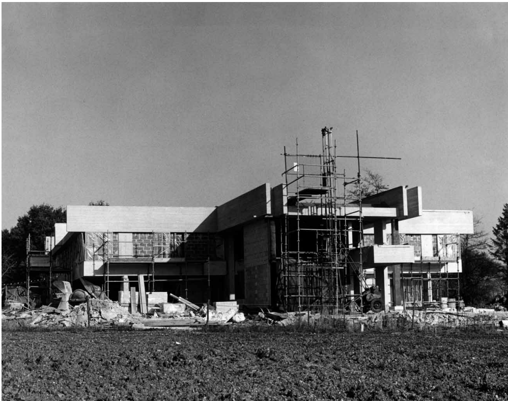
Figure 19. Hill House during construction, c. 1971. An ordinary quality of blockwork finishing can be seen on parts of the building which will soon disappear behind the highly refined surface blockwork, very light grey and laid with precision. (Lasdun Archive/RIBA Library Photographs Collection.)
