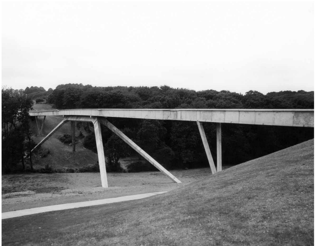
Figure 3. Whiteleigh Footbridge, Devon, Denys Lasdun of Drake & Lasdun, 1953–4 (demolished). Pre-stressed concrete engineering exploited, at this early stage in Lasdun's career, for visual effect. (Lasdun Archive/RIBA Library Photographs Collection.)
